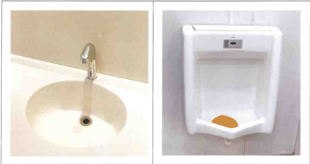
Photograph (2) & (3): Sensor based Taps and Urinals at MIAL terminal
