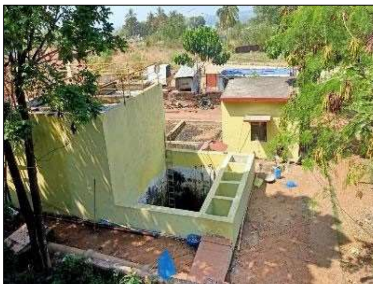
Photographs (1): Sewage Treatment Plant of 0.15 MLD under operation at MIAL
