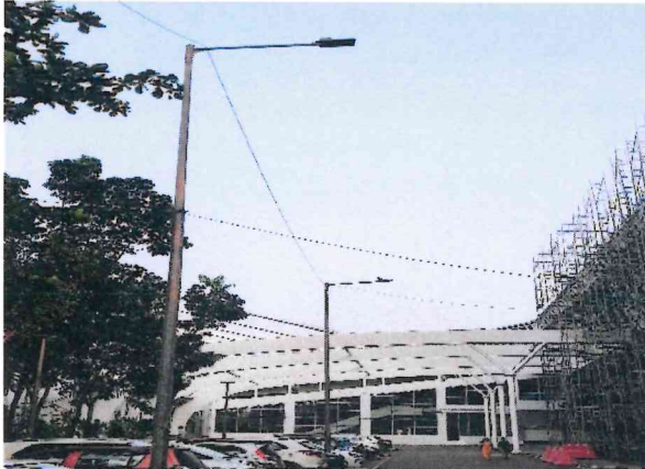
Street LED Lights
