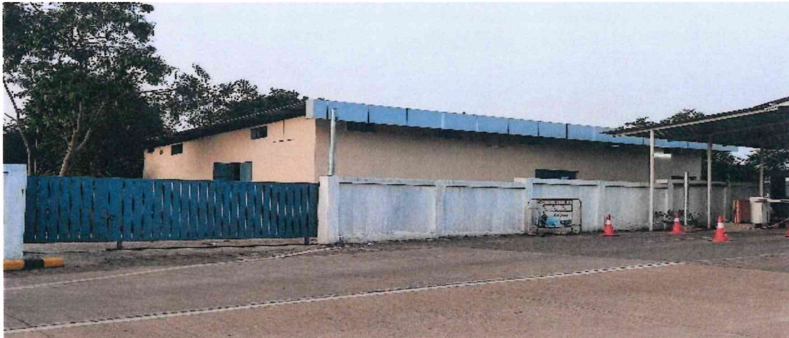
Waste Management Facility
